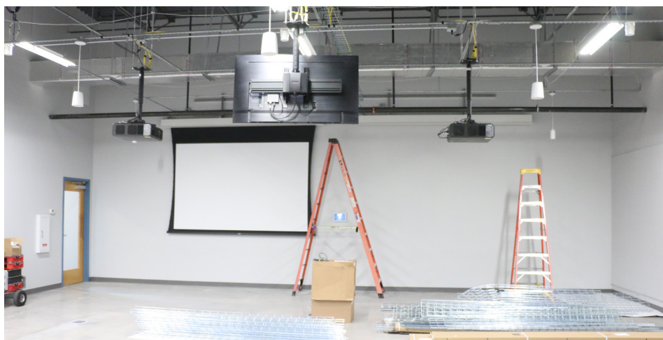
Learning Academy facility Da-Lite Advantage Projection ScreenChief projector mounts
